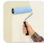
Apply paste to the wall ...
